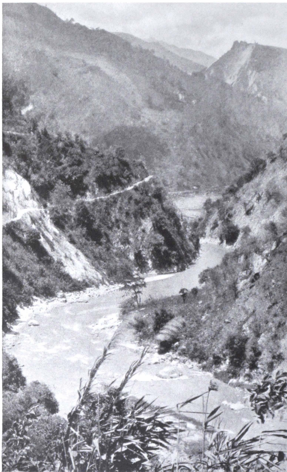
THE ROAD CUT OUT OF THE MOUNTAIN SIDE
